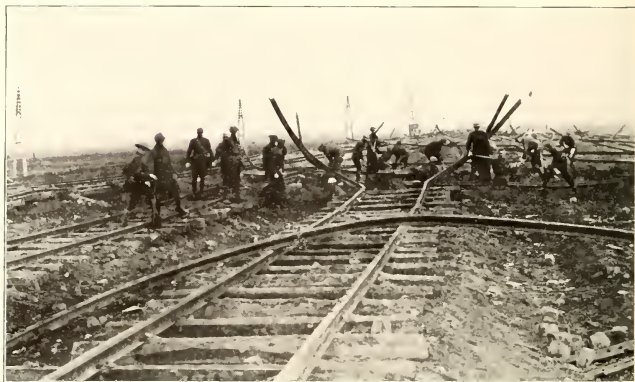
REPAIRING STANDARD-GAUGE RAILWAY DESTROYED BY THE ENEMY DURING THEIR RETREAT. IN THE FOREGROUND IS A MINE CRATER CAUSED BY A CHARGE PLACED BENEATH A SMALL CULVERT
